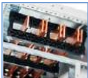
Linear busbar system: busbar system up to 3200 A positioned in the upper area.
