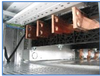
Linear busbar system: busbar system up to 3200 A positioned in the upper area.
