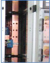
Sidebars: positioned in the left side area for the connection of the vacuum switch power clamps.
